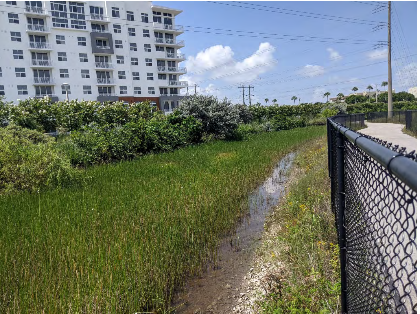
Buffer north of the Landmark South buildings continues to mature.
